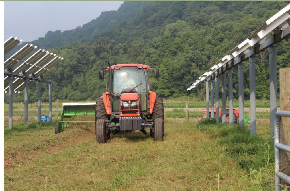
The dual land use pole and spline mounting system patented and installed by Hyperion Systems, LLC, Amherst, MA, demonstrates the possibility of baling hay between rows of solar panels on a farm in South Deerfield, MA.
