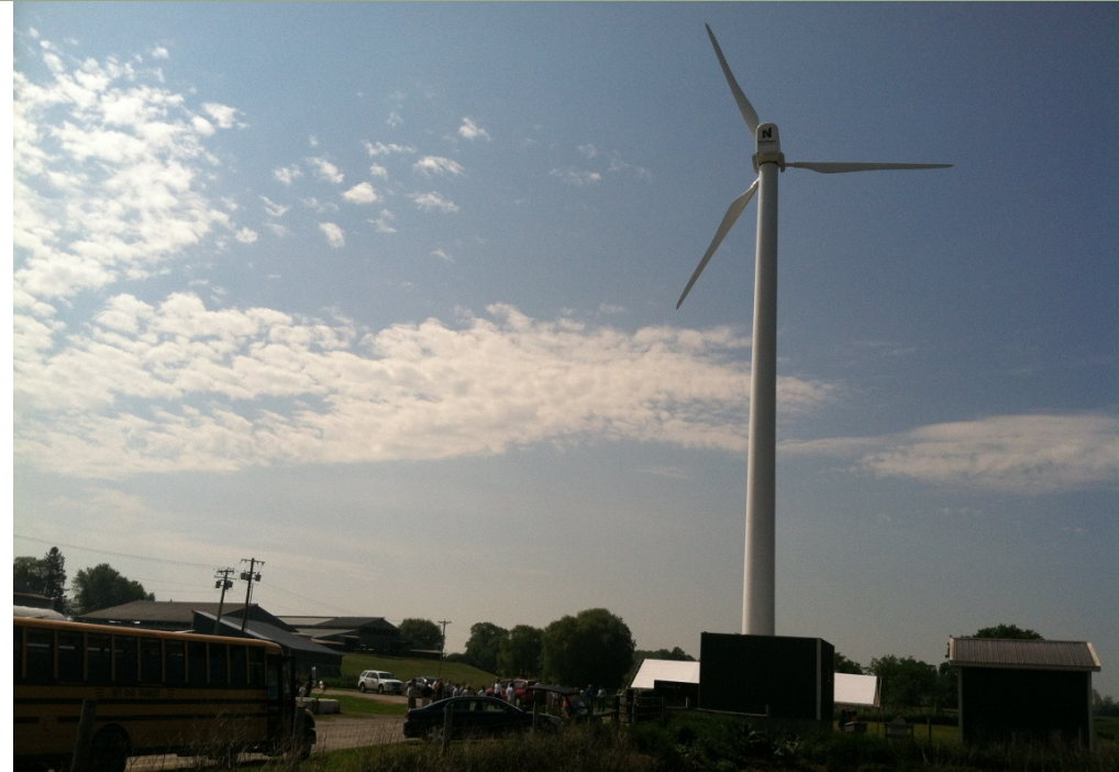
Just after Memorial Day in 2013, the Audet family hosted a community celebration of the installation of a 100-kilowatt wind turbine. A portion of the electrical output of the turbine is allocated to the local school.
