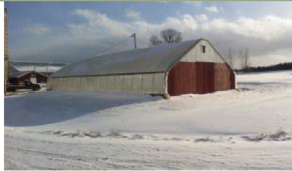
As the Maxwells worked with the system designers and equipment providers, they made sure to include heat recovery and distribution systems. The engine’s heat exchangers deliver heat for milkhouse water heating, for heat in the maintenance shop (saving 4-to-5 cords of wood or $800-$1,000 each winter), for the engine room, for drying separated manure solids, and for the greenhouse (pictured above).
