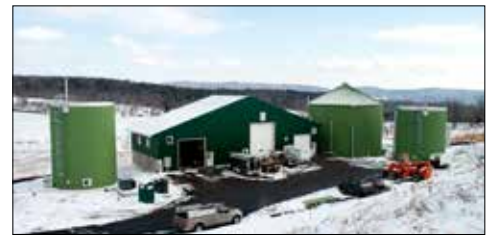
"Big Bertha" is Vermont Tech's community anaerobic digester, capable of generating 8,800 kWh per day.
